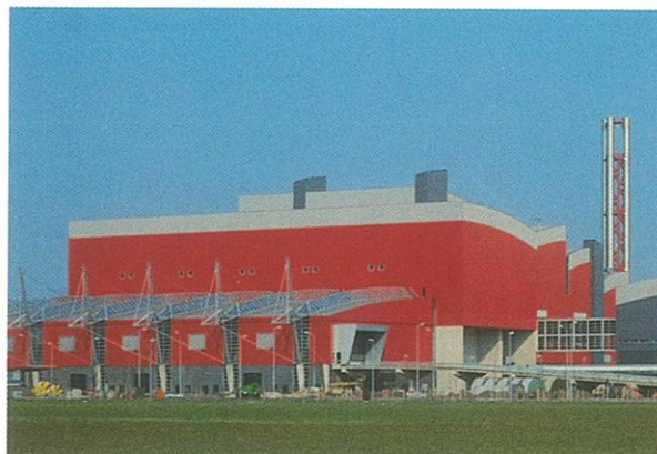
Gas engine feed water preheat of a waste-to-energy plant in Alkmaar, the Netherlands (3x W16V25SG)
