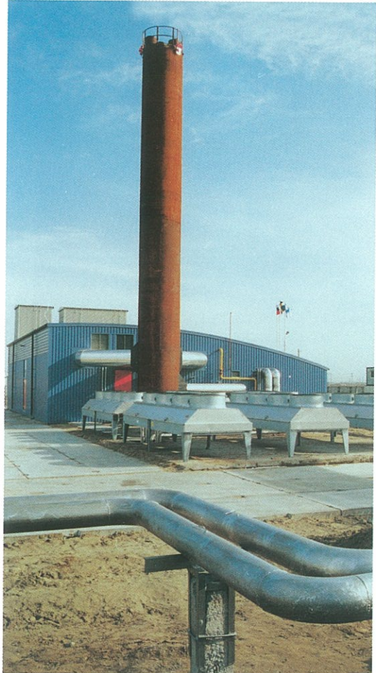
Modular built cogen plant in Tyumen, Russia (3xW16V25SG)
