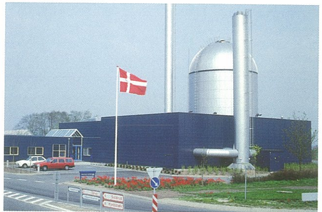
Municipal gas engine cogen plant in Støvring, Denmark (3xW16V25SG)
